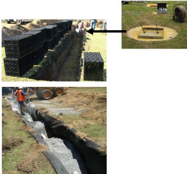
**Figure 3.** Installation of the two infiltration galleries in Floreat. The top left photo shows the Atlantis Leach System<sup>®</sup>, the bottom photo shows the gravel-filled gallery and the scored PVC pipe that distributed treated effluent to the ends of the gallery. The inspection points for viewing effluent inflow to each gallery are highlighted in the top right photo.
