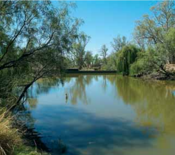
> Weir on the Condamine River Cecil Plains, Qld (MDBC)
