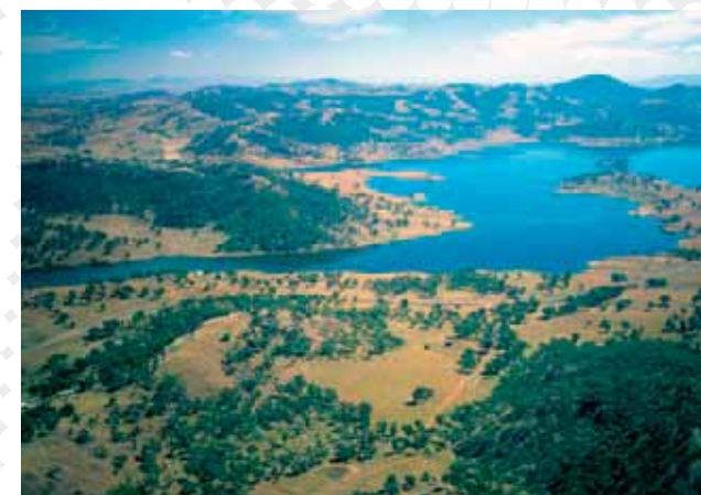
> Chaffey Dam, Namoi region, NSW (CSIRO)
