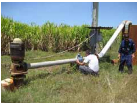
Installation of salinity and flow sensors
