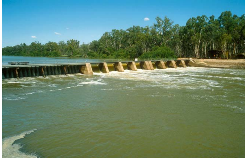
Figure 7. The location of weir structures, such as Lock 6, were used to determine the zone boundaries.
