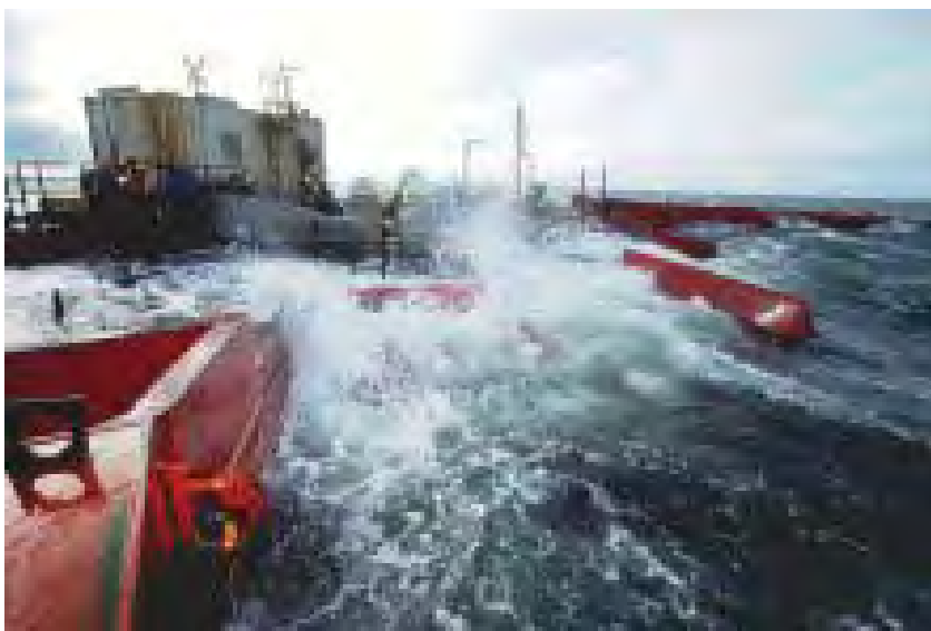
Figure 4-14 Wave Dragon prototype with an overtopping wave. Image courtesy of Wave Dragon [34].
