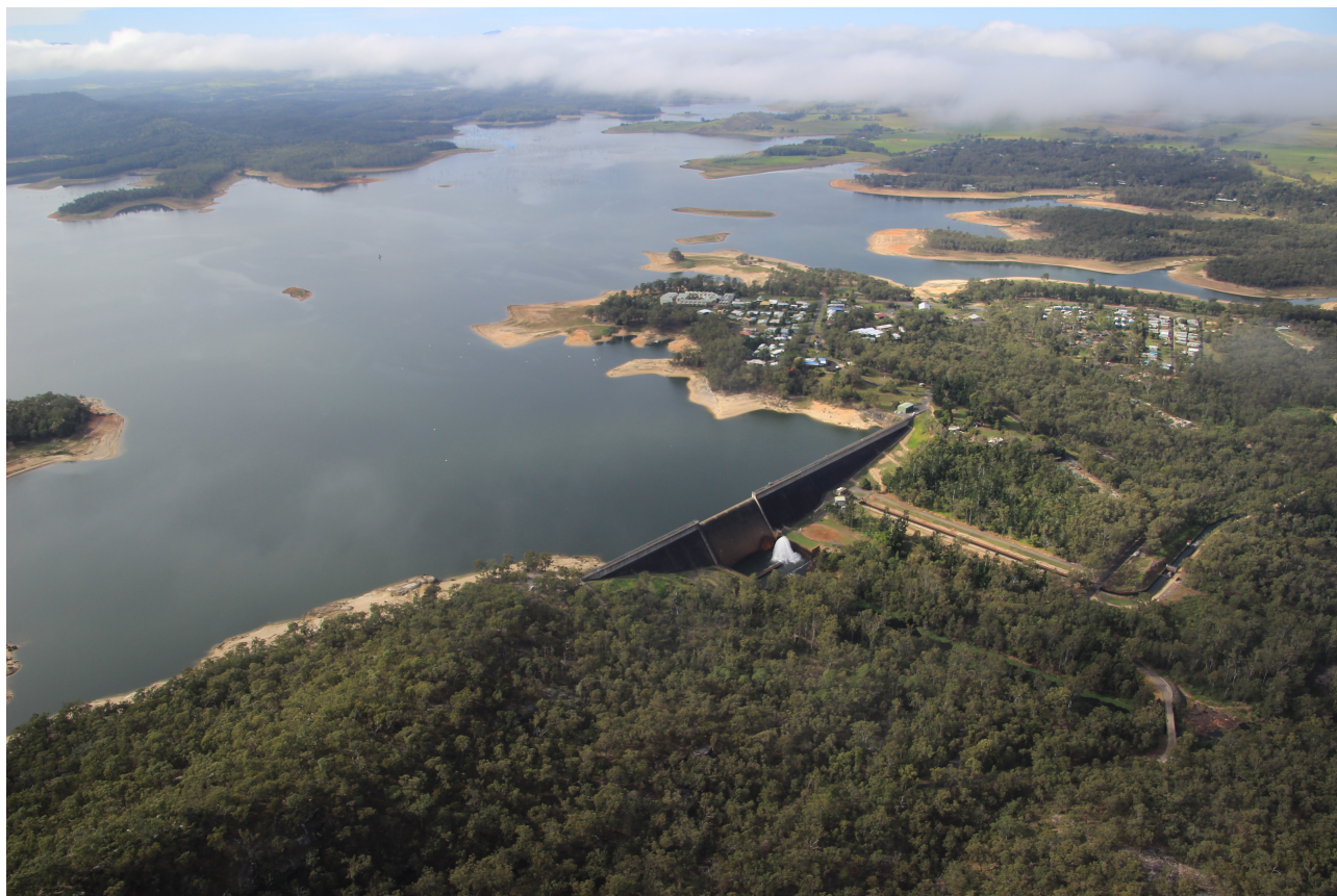
Figure 3-28 Tinaroo Falls Dam in the Barron catchment
