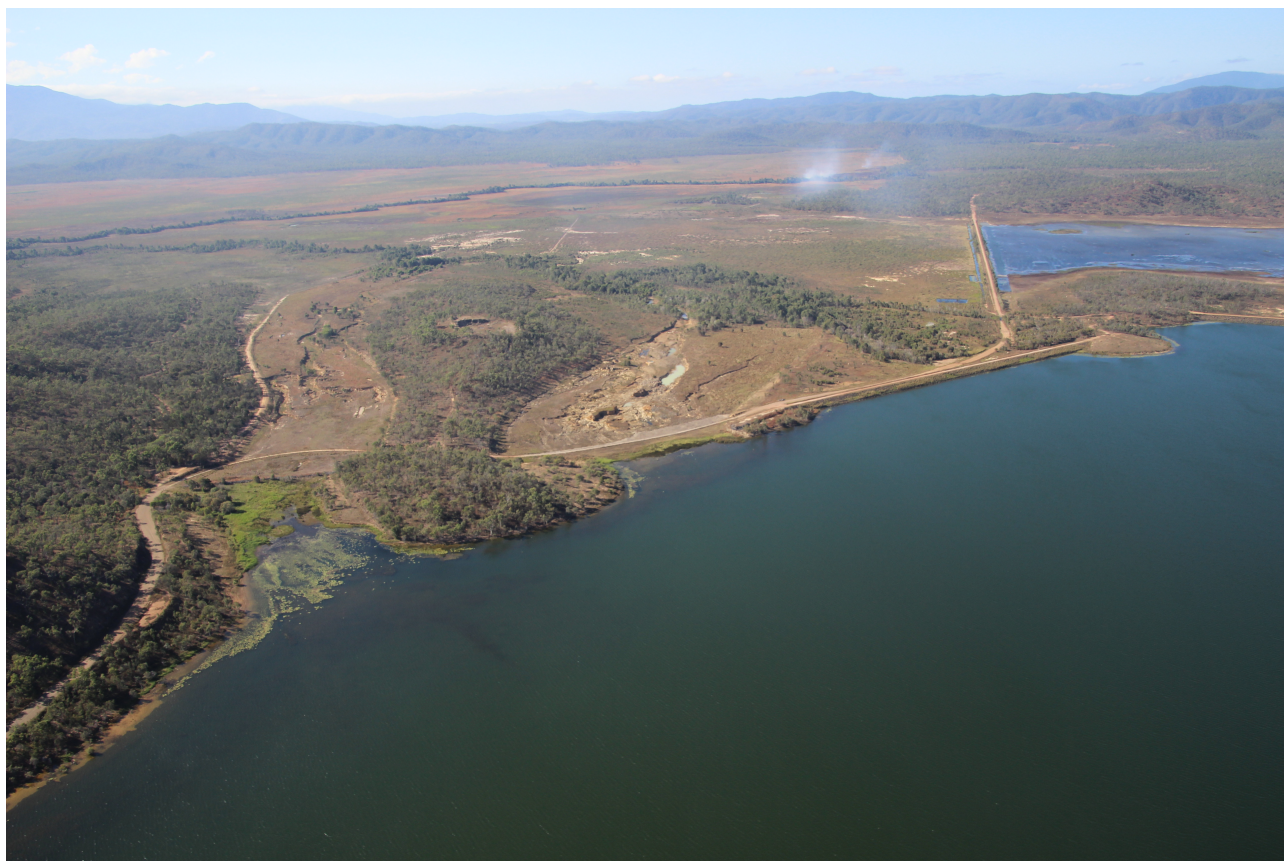
Figure 3-27 Main cross-river embankment of the Lake Mitchell Dam and spillways
