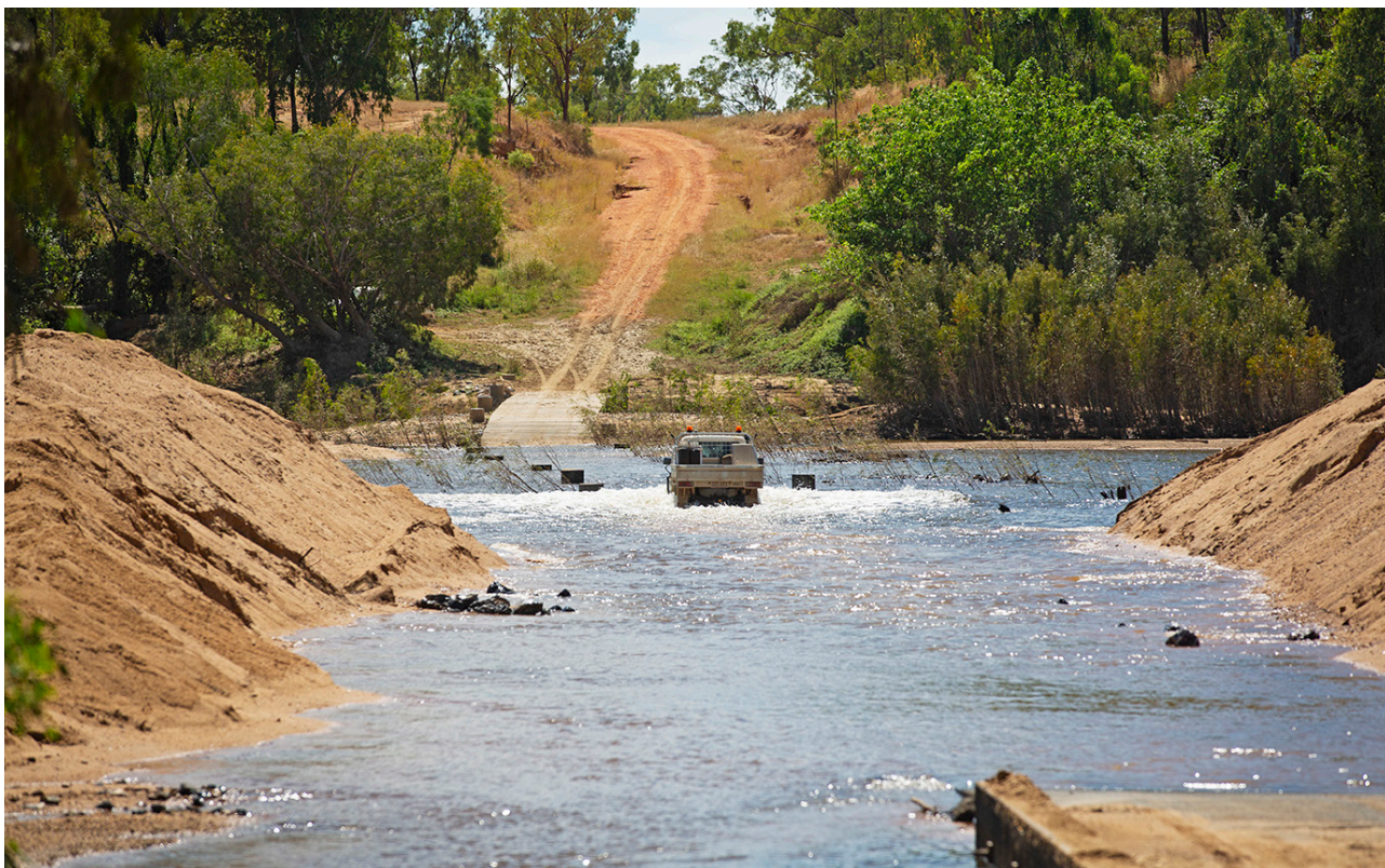
Figure 3-19 Creek crossings often have limited or no causeway and no bridge infrastructure
