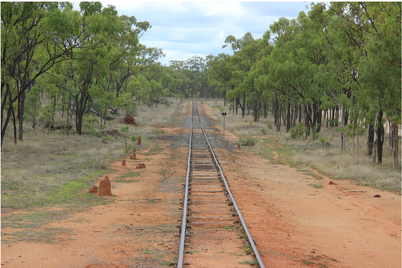
Figure 3-24 There is no rail infrastructure in the Mitchell catchment that can be used for freight transport Photo: CSIRO
