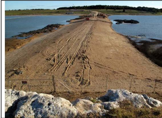
**Figure 11-11.** Main temporary flow regulator across the Goolwa Channel at Clayton Bay was completed in early August 2009 allowing water levels in the Goolwa Channel, Finniss River and Currency Creek to be raised and to saturate the existing exposed sulfuric material (map (c) in Figure 11-9). The regulator is about 400 metres long and 40 metres wide, and constructed as an earth-fill embankment.
