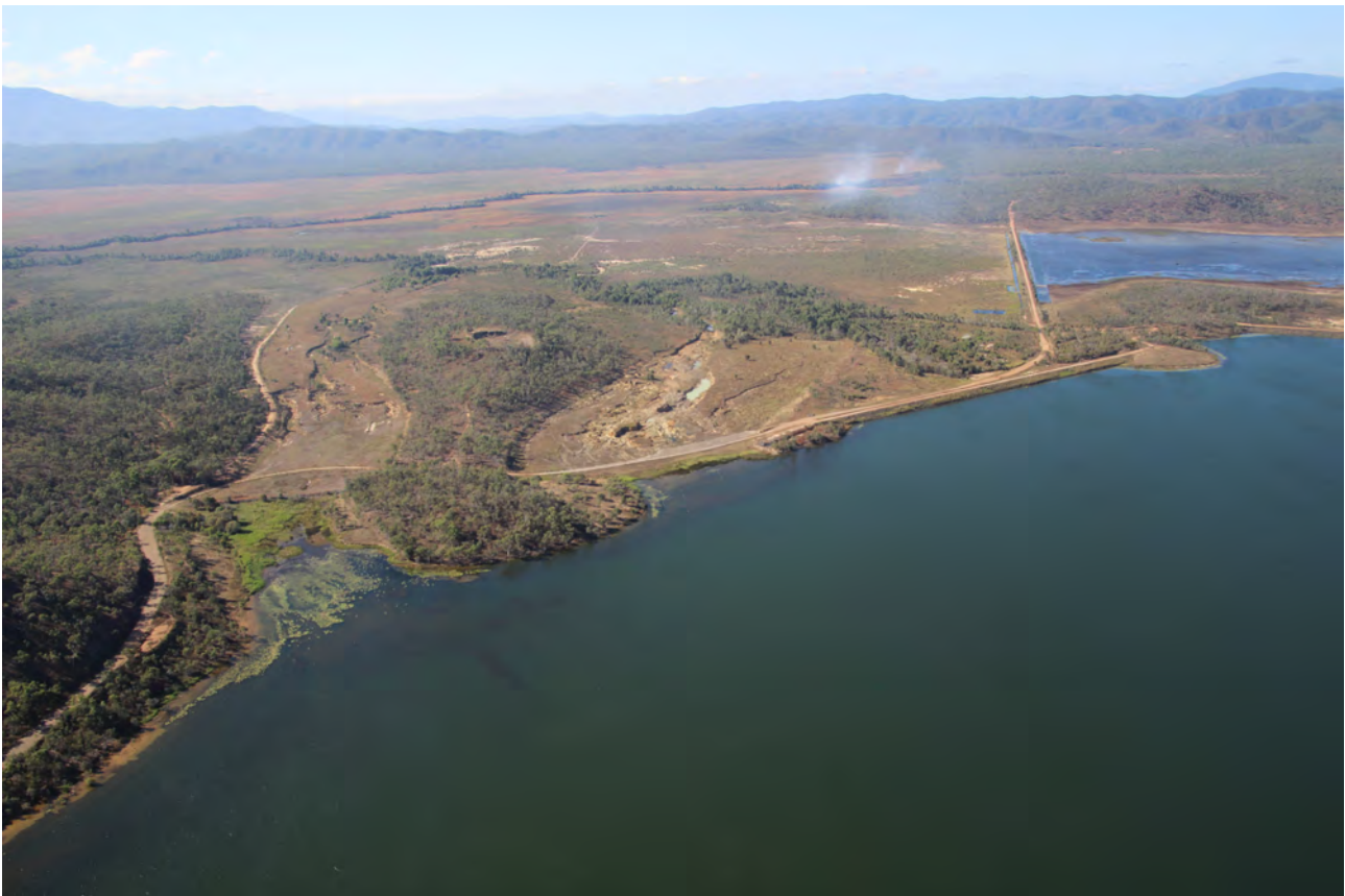
Apx Figure B-33 Lake Mitchell Dam looking downstream
