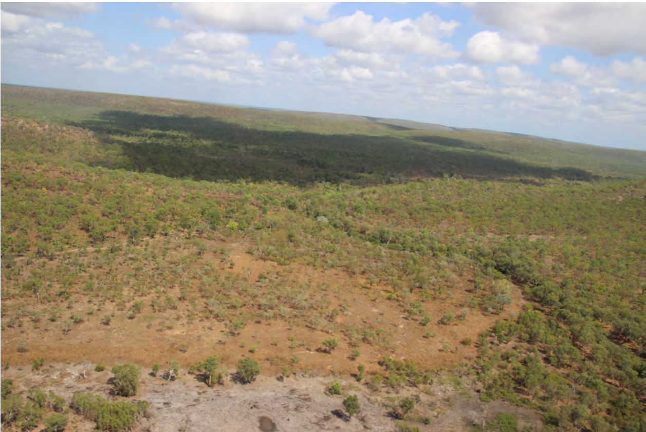
Apx Figure A-9 AROWS offstream storage looking upstream across the main axis
