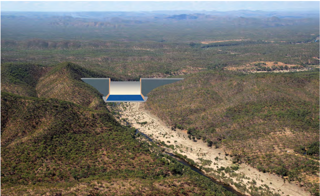
Apx Figure B-17 Palmer River dam site looking upstream
