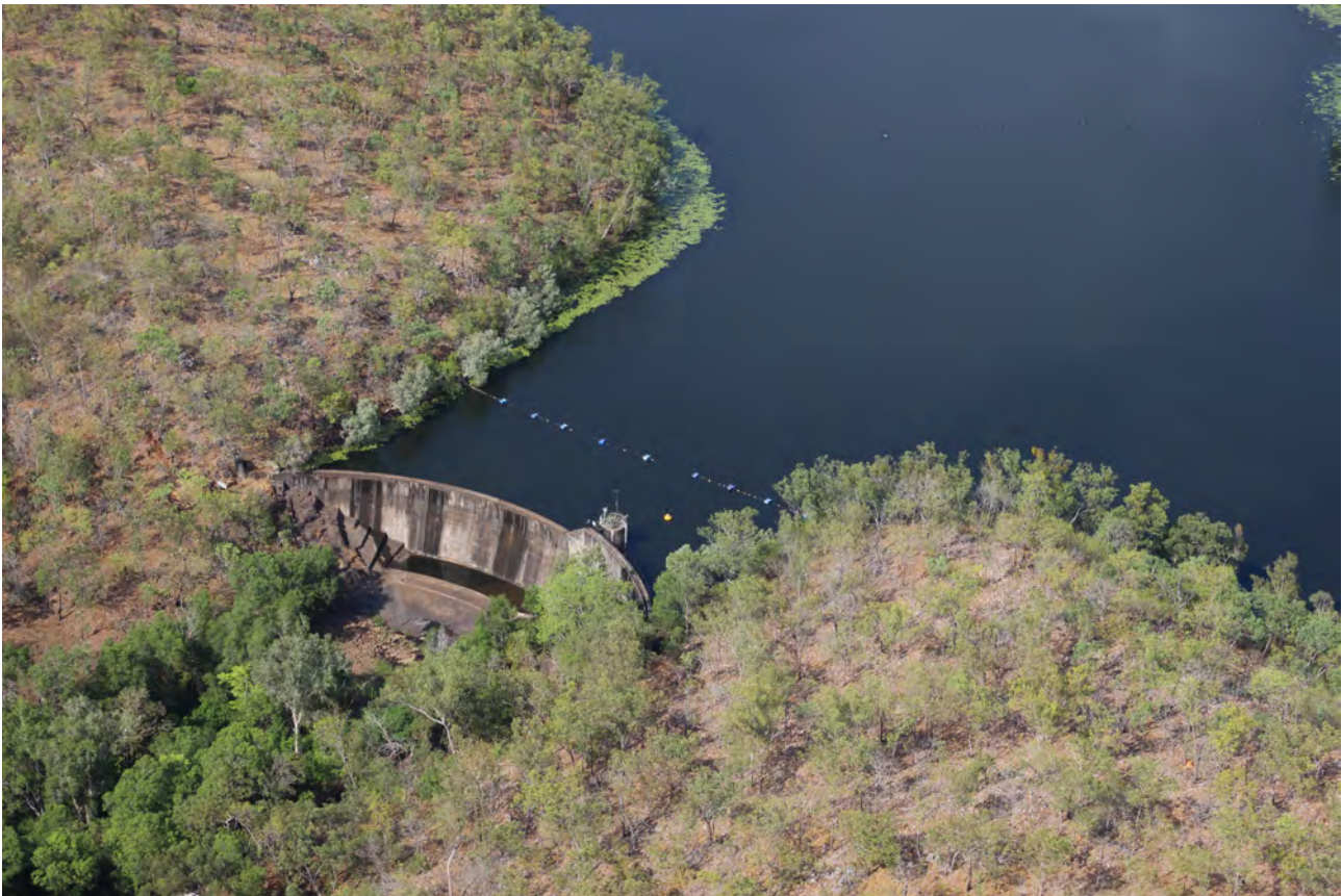
Apx Figure A-5 Manton Dam looking upstream
