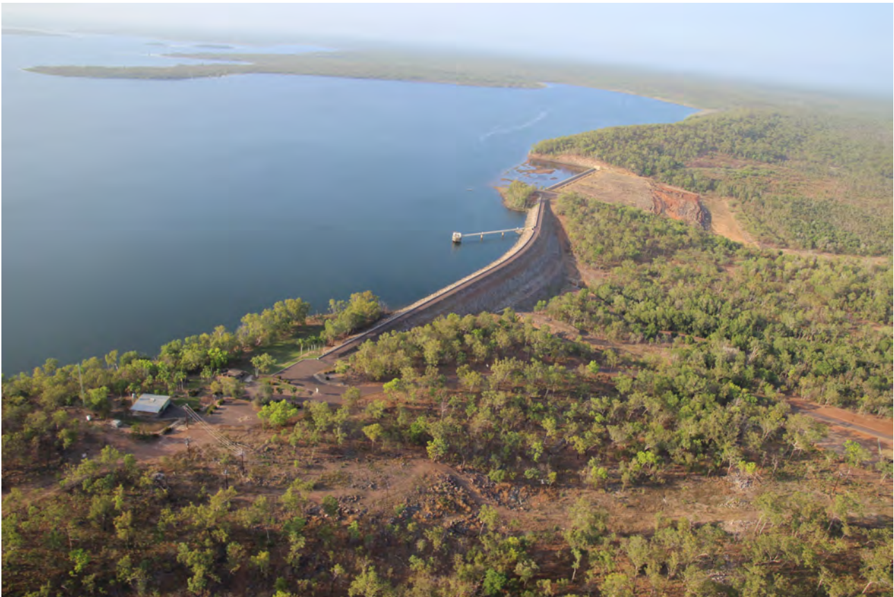
Apx Figure A-1 Darwin River Dam looking upstream
