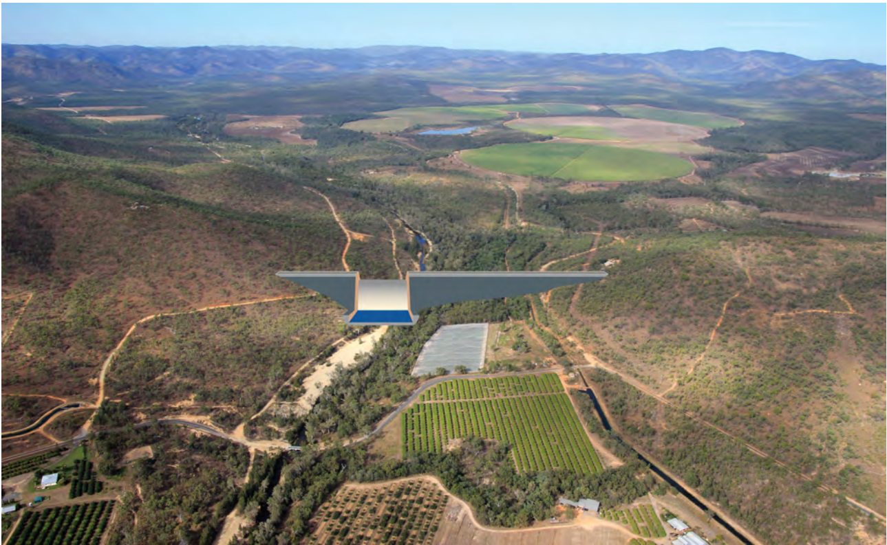
Apx Figure B-25 Nullinga dam site on the Walsh River looking upstream
