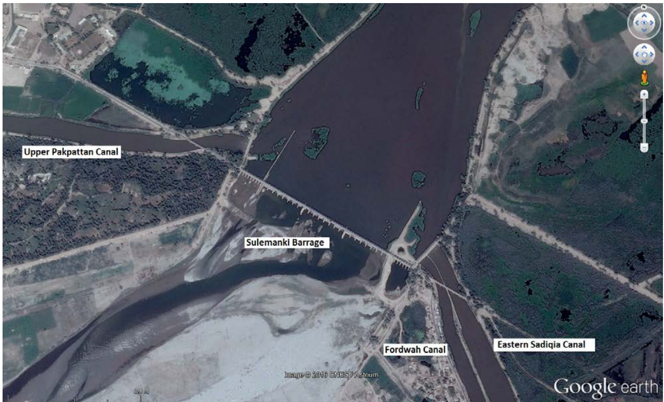
Figure 35 Sulemanki Barrage showing main barrage and offtake canals
