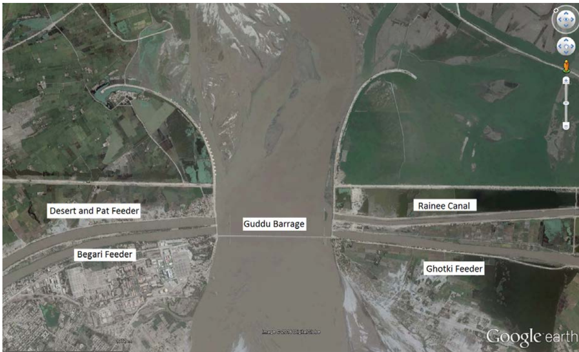
Figure 49 Guddu Barrage showing main barrage and offtakes
