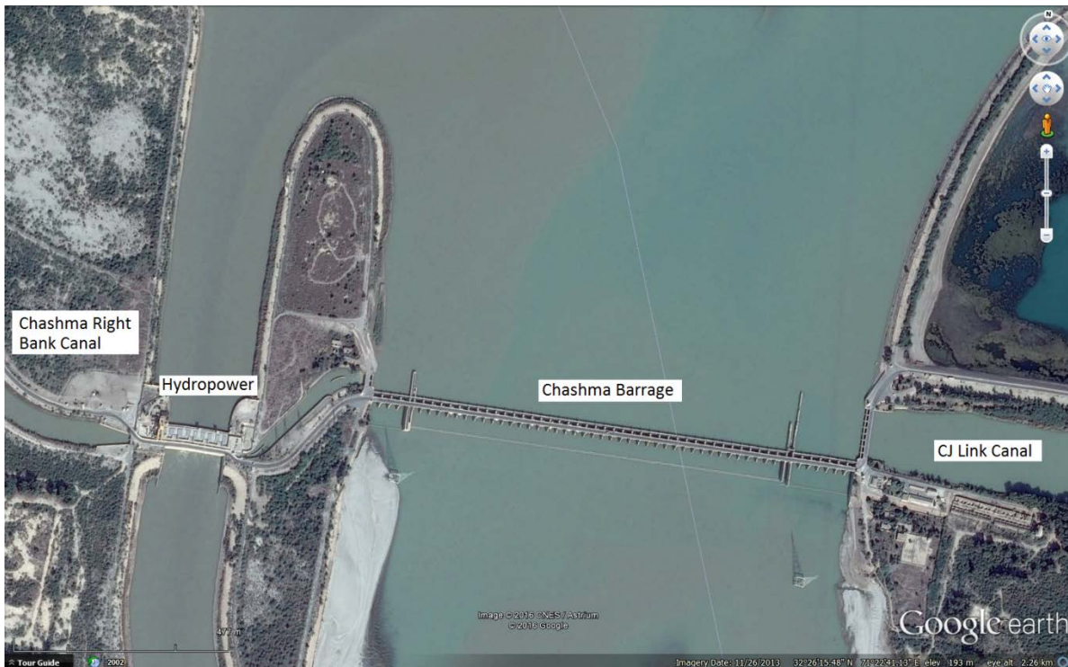
Figure 16 Chashma Barrage showing main barrage, hydropower and offtake canals
