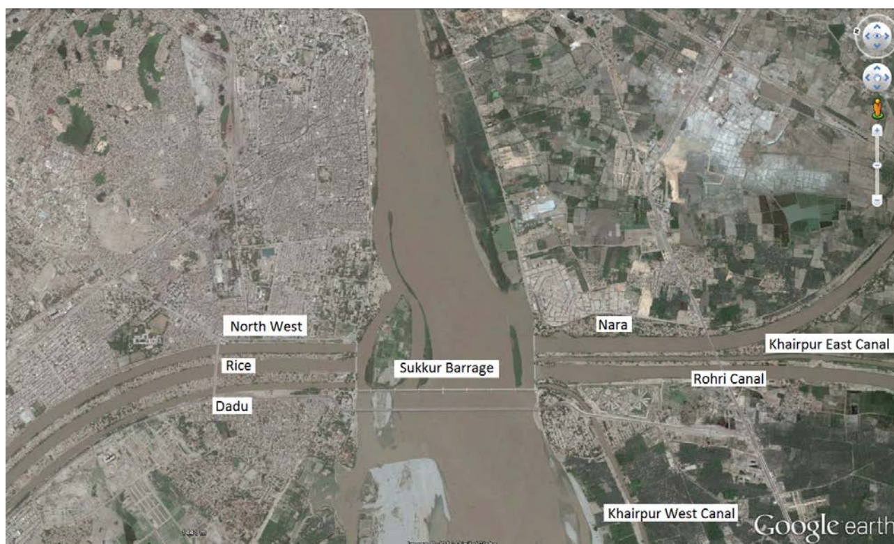
Figure 51 Sukkur Barrage showing main barrage and offtakes
