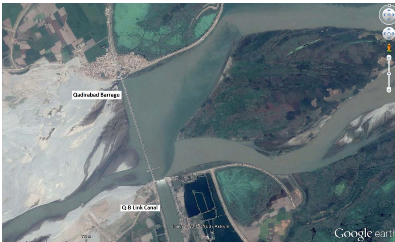
Figure 30 Qadirabad Barrage showing main barrage and offtake canal
