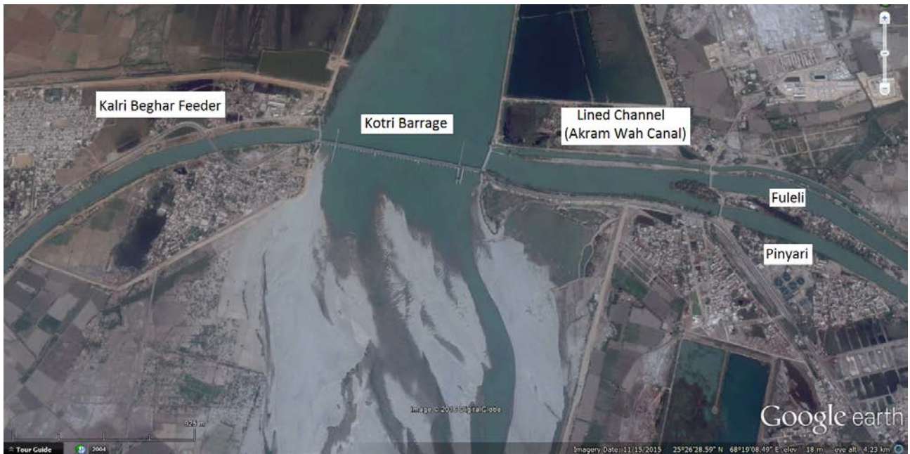
Figure 53 Kotri Barrage showing main barrage and offtakes
