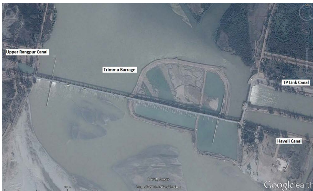
Figure 41 Trimmu Barrage showing main barrage and offtake canals
