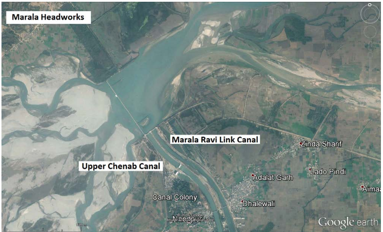
Figure 24 Marala Barrage showing main barrage and offtake canals
